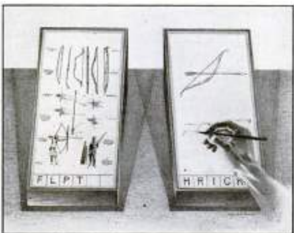
MEMEX IN USE is shown here. On one transparent screen the operator of the device writes notes and conceals dealing with reference material which is projected on the screen at left. Insertion of the proper code symbols at the bottom of right-hand screen will tie the new items to the earlier one after notes are photographed on supermicrofilm.
